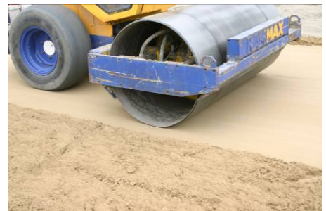
Compaction by roller.
