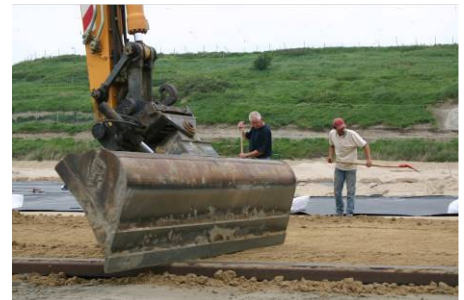
Determining layer thickness made easy by using a steel height beam.
