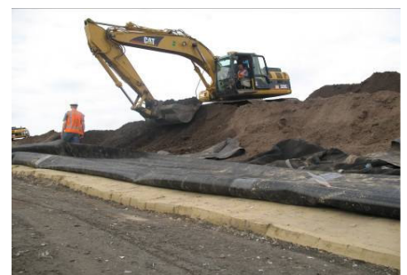
Trisoplast is covered by HDPE foil, geotextile and drainage layer.
