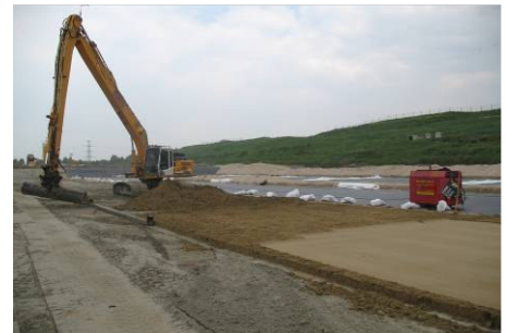
Application and compaction of the mixture.
