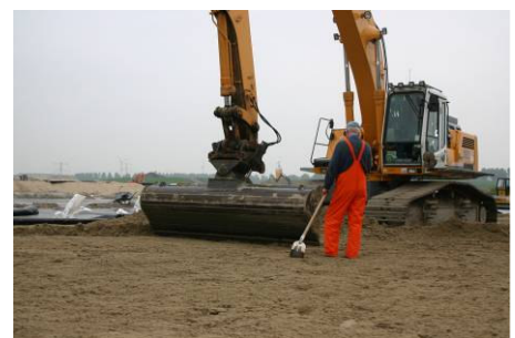
Measuring the layer thickness manually.
