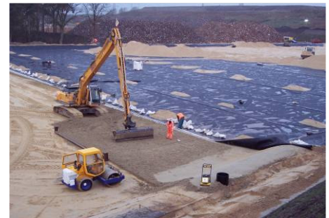
Compaction of the layer done by both roller and vibrating plate.
