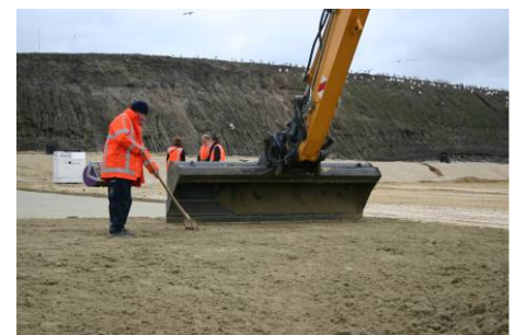
Checking layer thickness manually.
