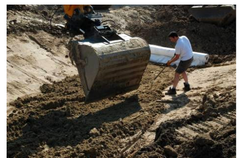
Manual layer thickness check.
