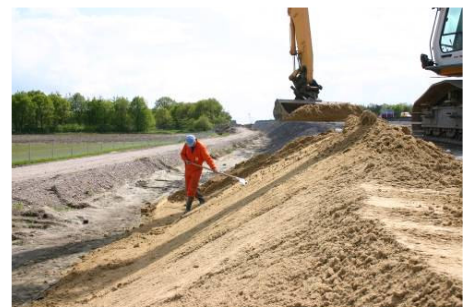
Installation on slopes.
