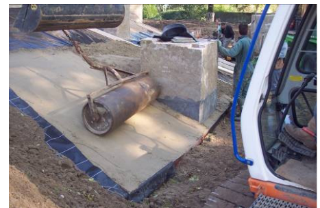
Trisoplast compaction on slopes.
