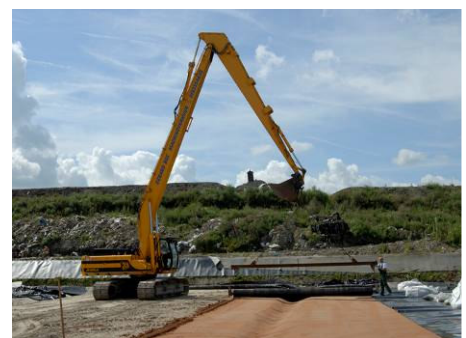
Covering the Trisoplast layer with HDPE geo-membrane.
