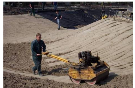
Compaction of the Trisoplast.
