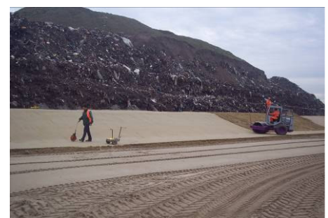
Quality control after compaction.
