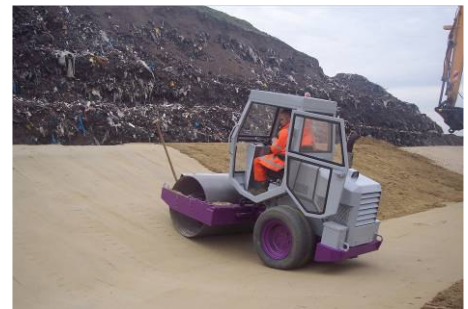
Compaction of the newly applied Trisoplast layer.
