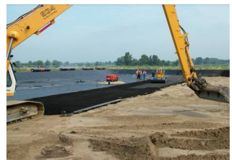
Application and compaction of Trisoplast.
