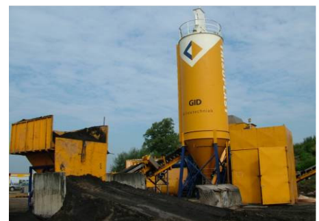
Mobile mixing plant installed at project location.
